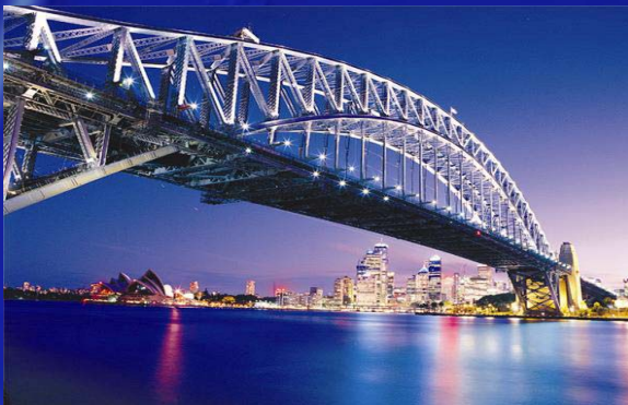
Bridge and Building Monitoring
