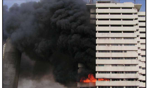
Building Fire Detection
