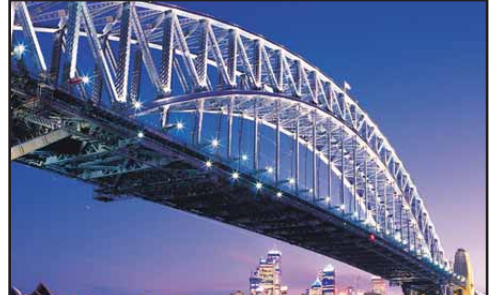
Bridge and Building Monitoring
