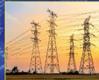
Power Line Monitoring
