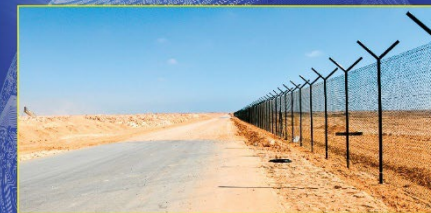
Border Security Monitoring
