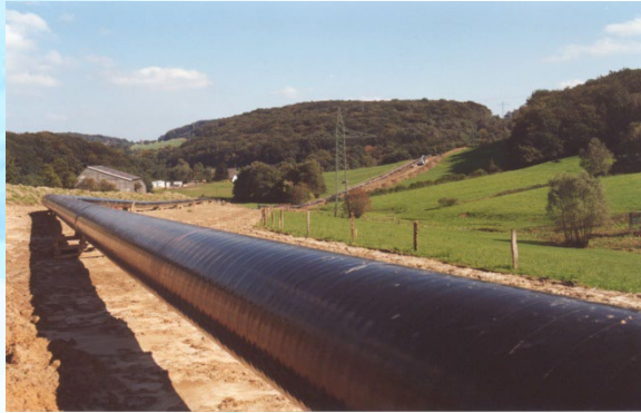
Oil and Gas Pipeline Monitoring
