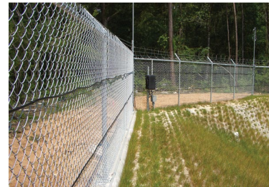
Border Security Monitoring
