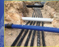
Underground Power Line Monitoring
