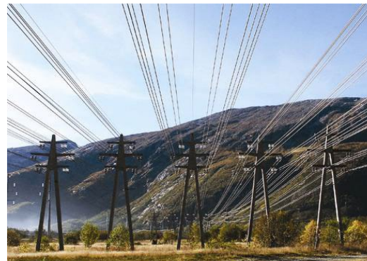
Power Line Monitoring
