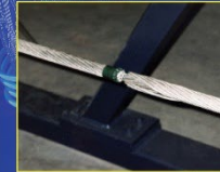
Optical Ground Wire (OPGW)
