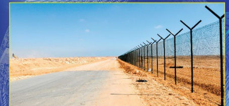
Border Security Monitoring
