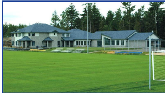
Training Centre Building
