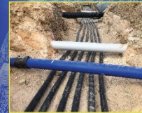
Underground Power Line Monitoring
