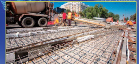
Highway Health Monitoring
