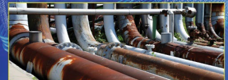
Corrosion and Erosion Monitoring
