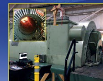
Gas Generator Monitoring
