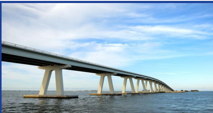
Bridge and Building Monitoring
