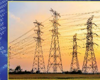
Power Line Monitoring
