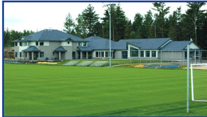
Training Centre Building
