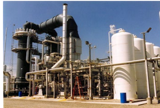
Steam Plant Monitoring
