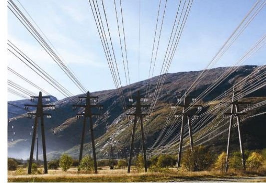
Power Line Monitoring
