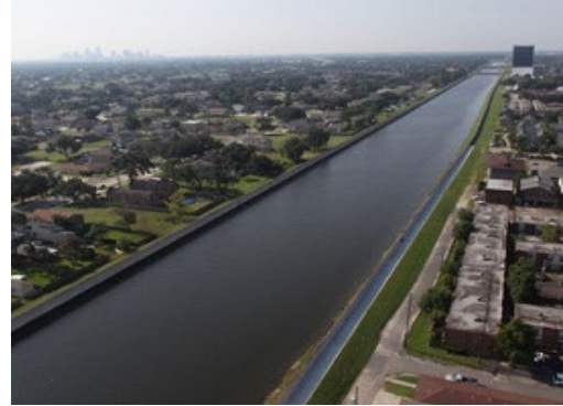
Dam and Levee Monitoring
