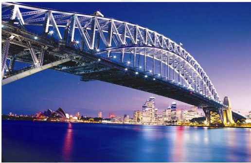
Bridge and Building Monitoring
