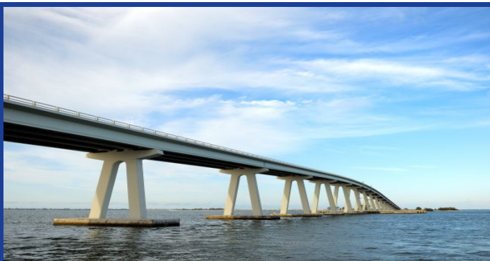
Bridge and Building Monitoring
