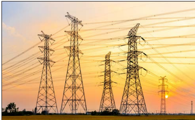
Overhead Power Line Monitoring
