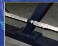
Optical Ground Wire (OPGW)
