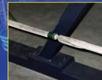
Optical Ground Wire (OPGW)
